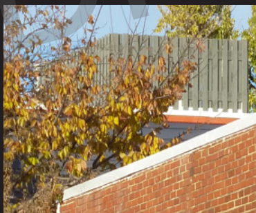
Example of appropriate roof-mounted HVAC screening.
